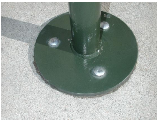
Example of baseplate - note the vandal resistant fasteners used to anchor the rack. (photo courtesy James Mackay, City of Denver)
